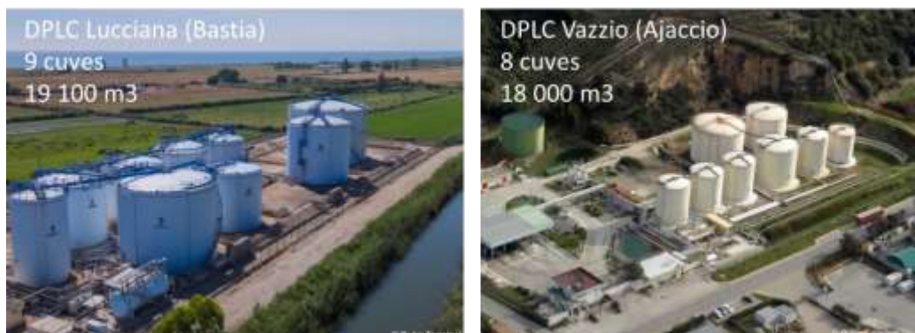
Figure 10 - Sites de stockage de DPLC (source : Rubis terminal)
